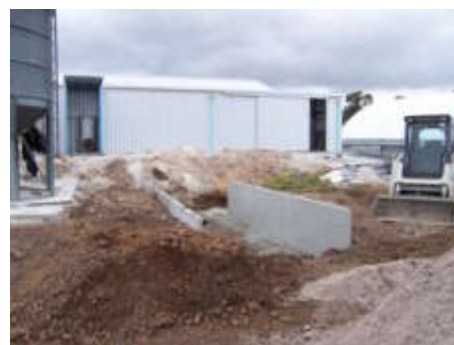
Works on the trafficable sump
